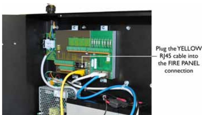
Figure 2.21 — C2CN Fire Panel Connection details
