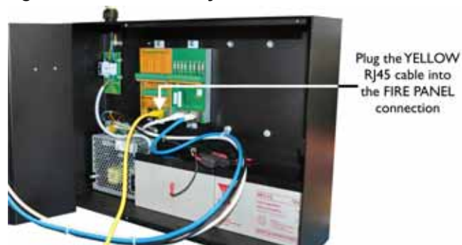
Figure 2.13 — Yellow RJ45 Cable connected to C2CFPE
